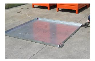
Lay the first paving element on the ground and place the spacers (at least 2 per contact side).
