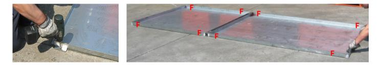
Secure the flooring elements to the ground using the fixing elements. The fixing elements (F) are placed only on the outer perimeter.
