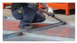
Cover the joints using the junction elements.
