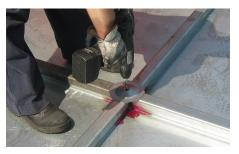
At the intersection (if there are 4 flooring elements) put the cross element and fix it to the ground.
