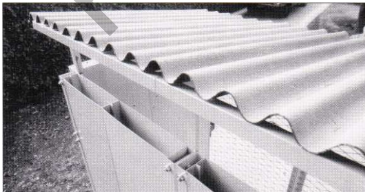
Tettuccio ondulina in cartone catramato - Tarred corrugated boarti roof
